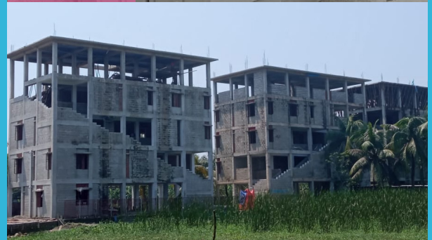
UNDP NUPRP's affordable housing in Noakhali District, with 102 units.
