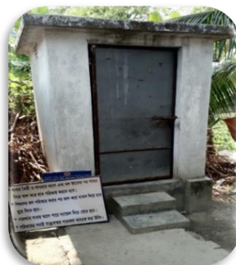
Image 3.19 Latrine Facility, Town Jainkathi CDC, Patuakhali Municipality
