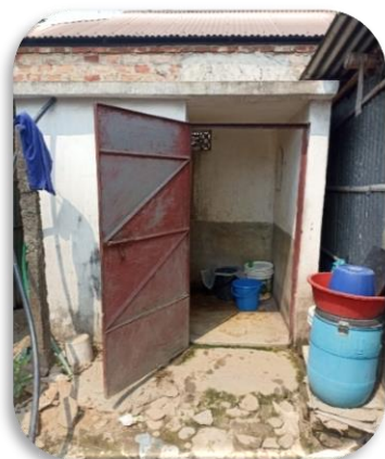
Image 3.15 Bathroom Facility, Lama Para CDC, Sylhet City Corporation
