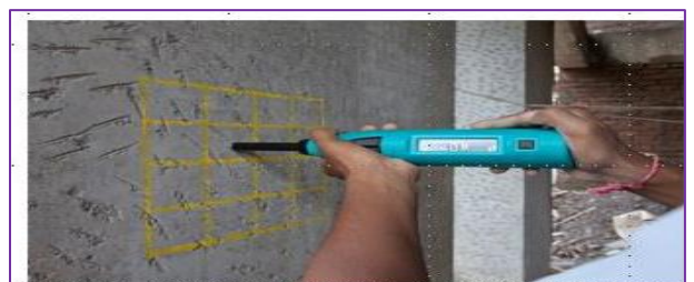
Hammer / rebound test
