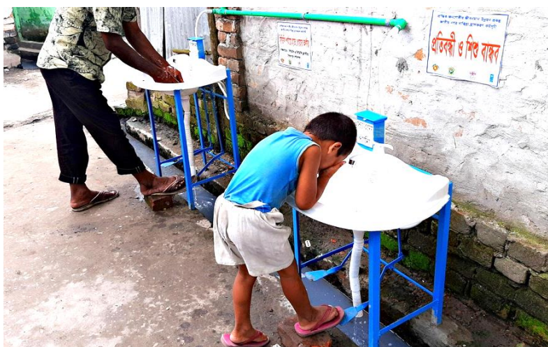
Innovative hand washing basins with leg pedal set up especially for people with disability & children at Saidpur Paurashava PC: Md. Mostafizur Rahman
